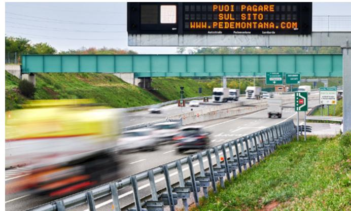
1. **the detection systems** located on the portals **identify the onboard device via radio** for the purpose of **charging the toll** in accordance with the terms and conditions of the contract between the customer and the third-party company providing the payment service
